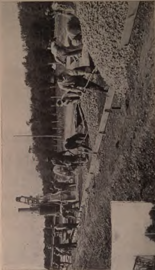
The road here illustrated as under construction is known as the Pacific highway, and is located in Lewis county, Wash. It is being laid in two courses, the base being of a 1:3:6 mixture with egg gravel, 5 inches thick at the center and 3½ inches at the sides. The surface is a 1:1:2 mixture with pea gravel. The width is 16 feet. A Koehring street paving mixer is being used.
